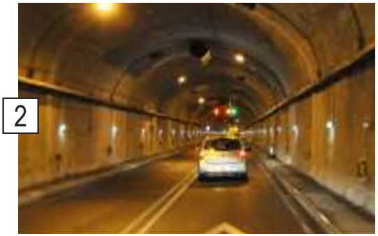
2 Tunnel de Bielsa/Aragnouet
